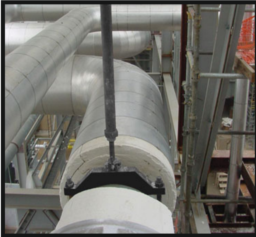
Rigid Strut with Fig RY3 stiff clamp
